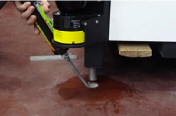
Figure 3.12. Fill the holes with chemical resin
