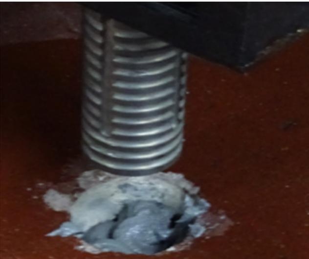
Figure 3.13. Chemical resin in drilled holes
