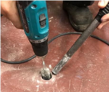
Figure 3.4. Cleaning drilled holes
