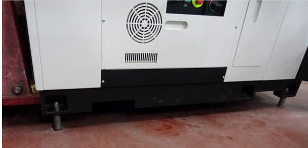
Figure 3.9. Verify the drilled holes through prepositioning
